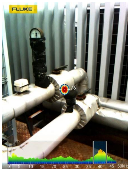
Leak detection on a pipeline
